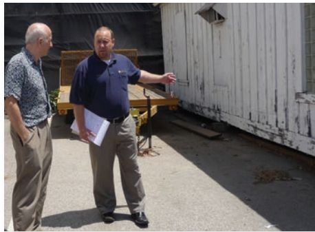
Reuben Lombardo of Spectra Corporation (on right) discusses rehabilitation of the original board and batten walls with Project Architect Mario Fonda-Bonardi.
