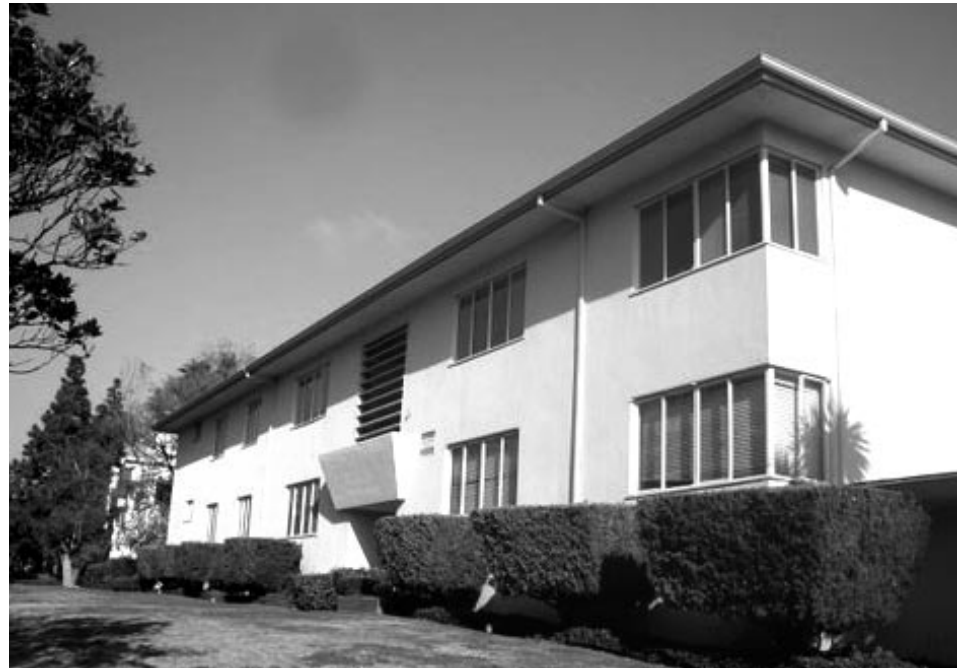
Landmark Status Given to Teriton Apartments.
