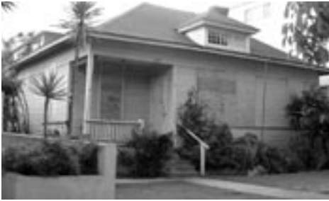
New landmark at 1012 Second Street
