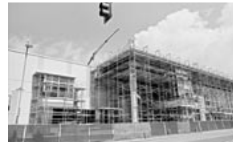
Construction of the new Main Library, 601 Santa Monica Blvd. photographed by Cynni Murphy, March 28, 2005 (Santa Monica Public Library Image Archives #M235)
