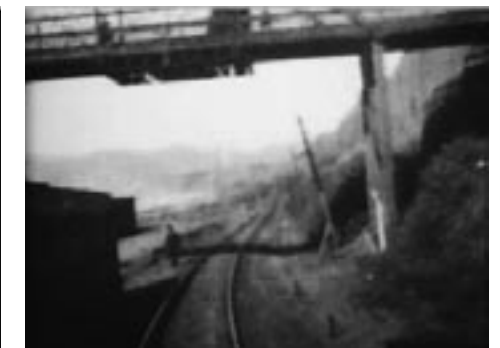
Heading north up the coast from the tunnel, the tracks follow the path of today's Pacific Coast Hwy. with the distinctive cliff towering above on the right.
